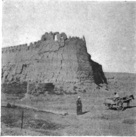
THE WALLS OF BOKARA
